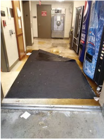
Liquid from biohazardous waste bags sprayed from an autoclave into a hallway at the University of North Carolina, Chapel Hill. A clogged drain/strainer was a partial cause (photos courtesy of UNC EHS).
